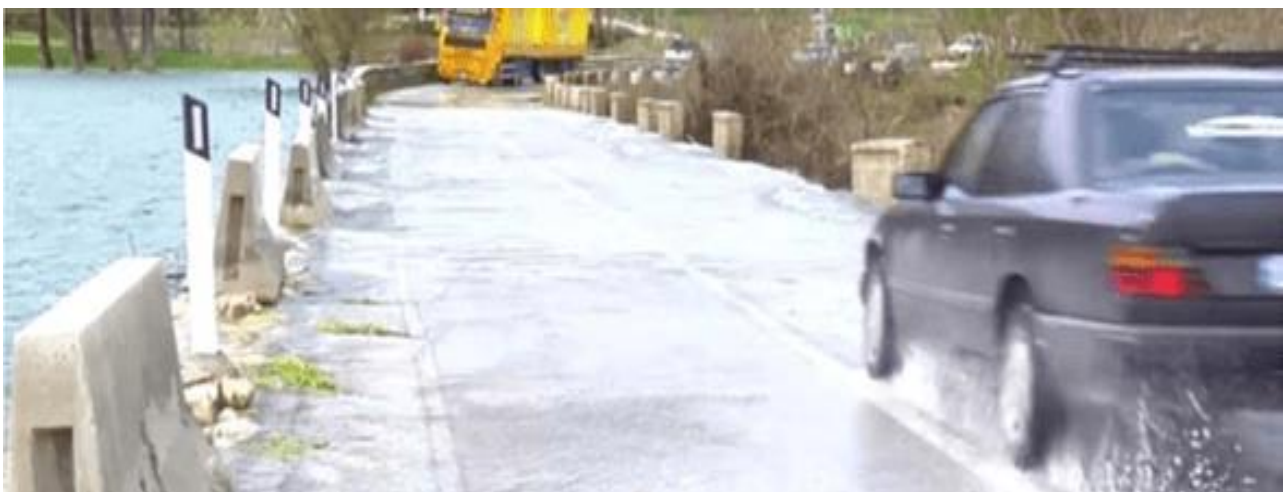
Figure 1: Lake Viroi water level over the road segment and the bridge
