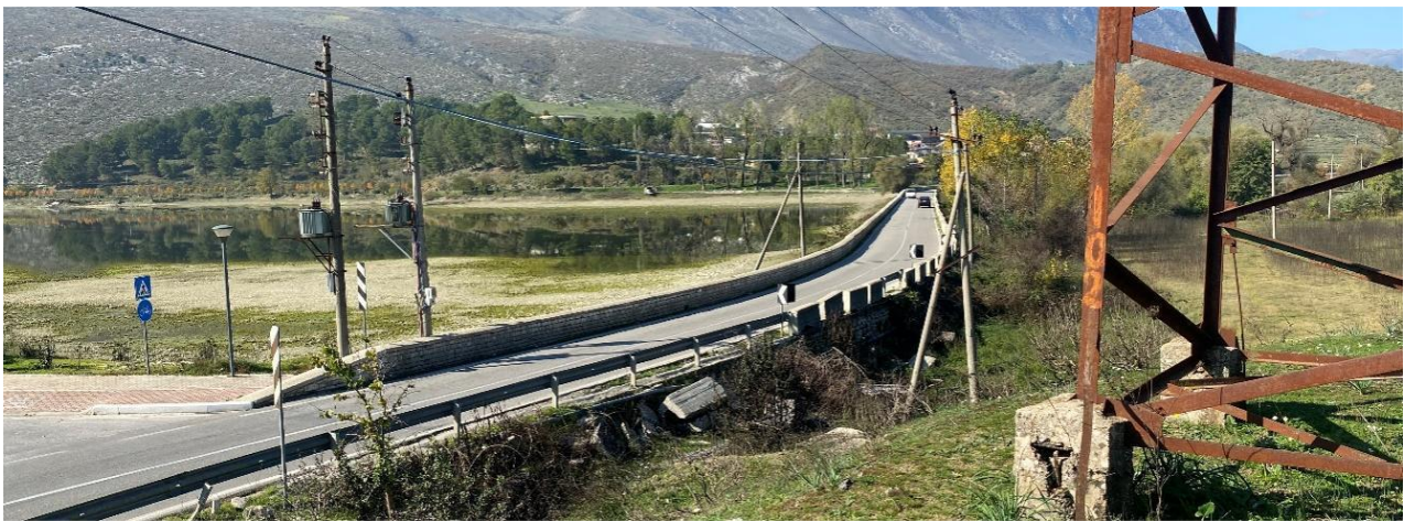
Figure 4: Overview of the Existing Road and Bridge
